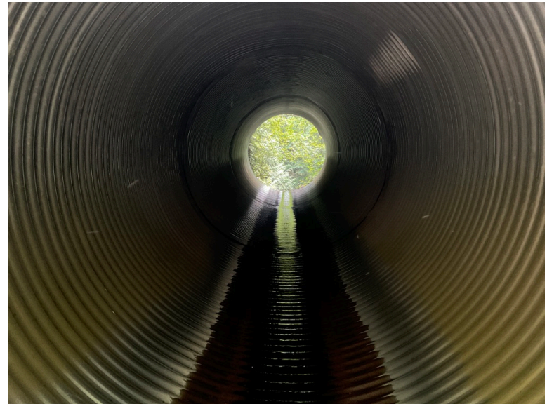
Looking Downstream Through CMP
